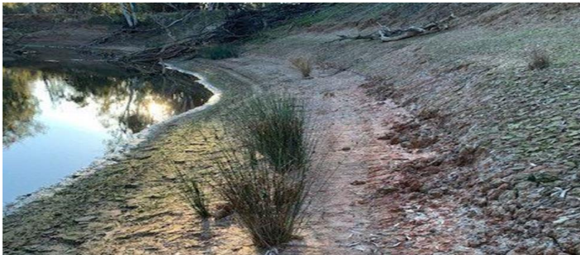
Figure 2: Evidence of erosion, notching and loss of bank on the Lower Goulburn
