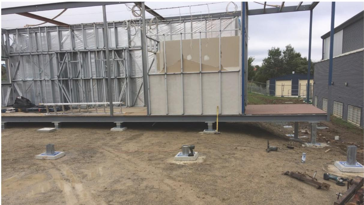
**Site footings prepared, checked and ready to receive further modules** [Credit KLMS]
