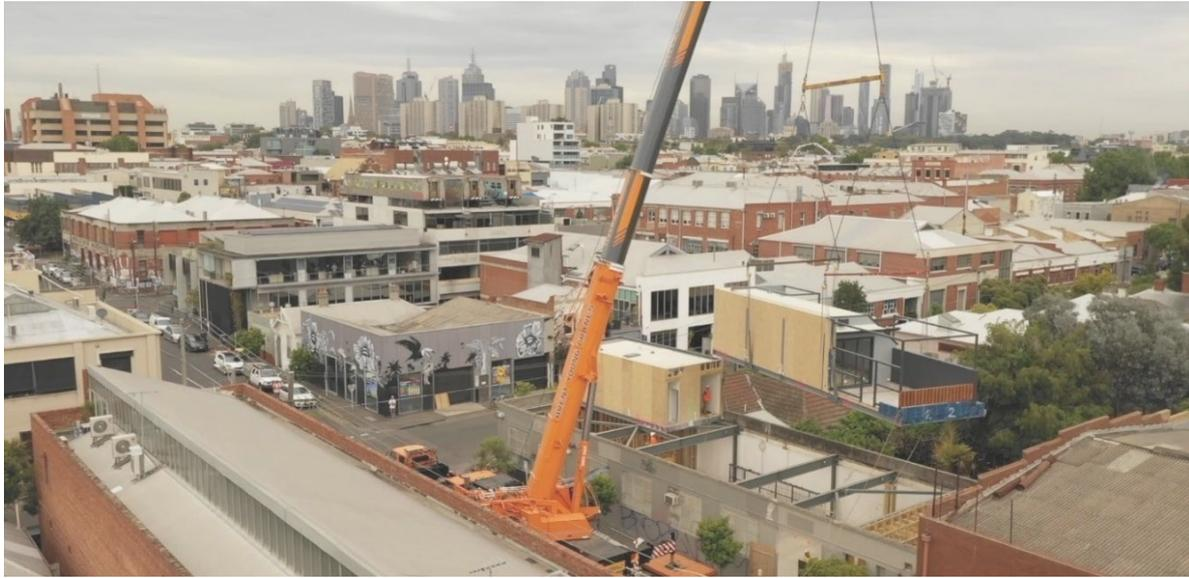
**Module installation with specialised rigging in a tight environment** [Credit XXX]
