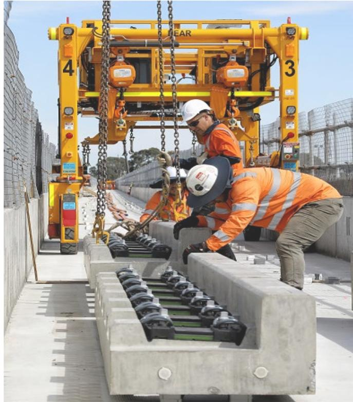
**Specialist designed lifting system for handling prefabricated rail precast components** [Credit LXRP]
