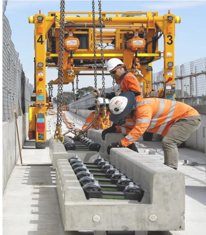
**Specialist designed lifting system for handling prefabricated rail precast components** [Credit LXP]
