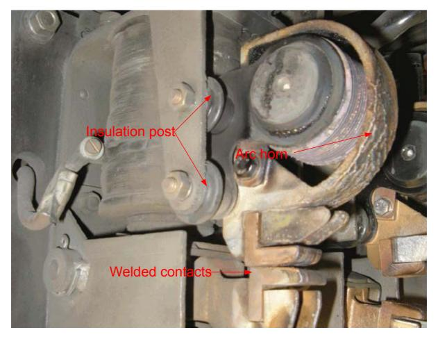
Figure 13 – Grouping contactor LS1
