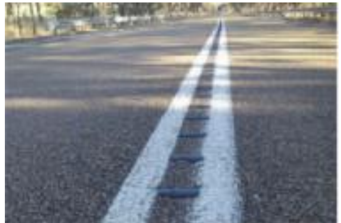
Figure 2: Audio tactile line marking (ATLM)
