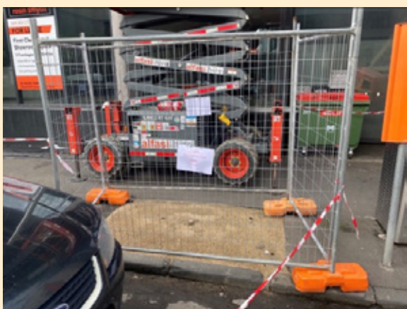
Image: Temporary fencing and signage indicating the ‘Tree Protection Zone’ in Example 1.
