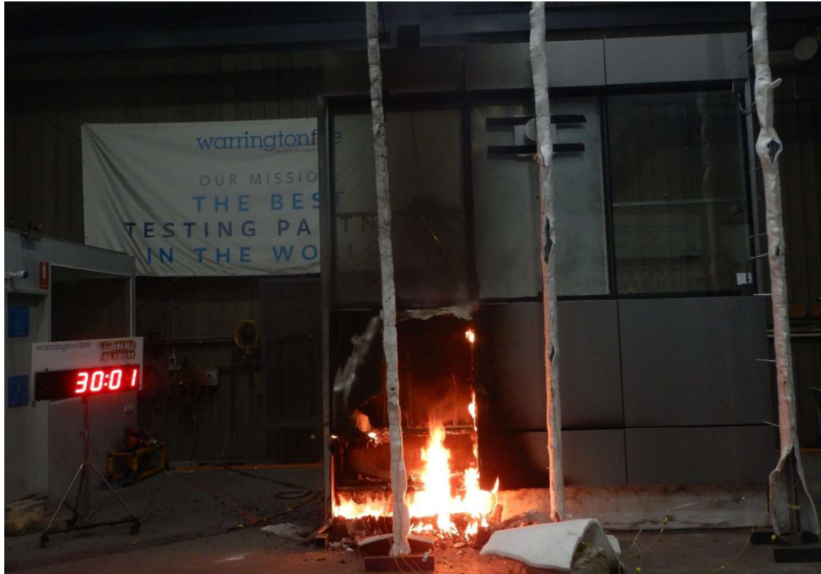
Figure 36 The specimen 30 minutes (1 second) into the test - burner turned off.
