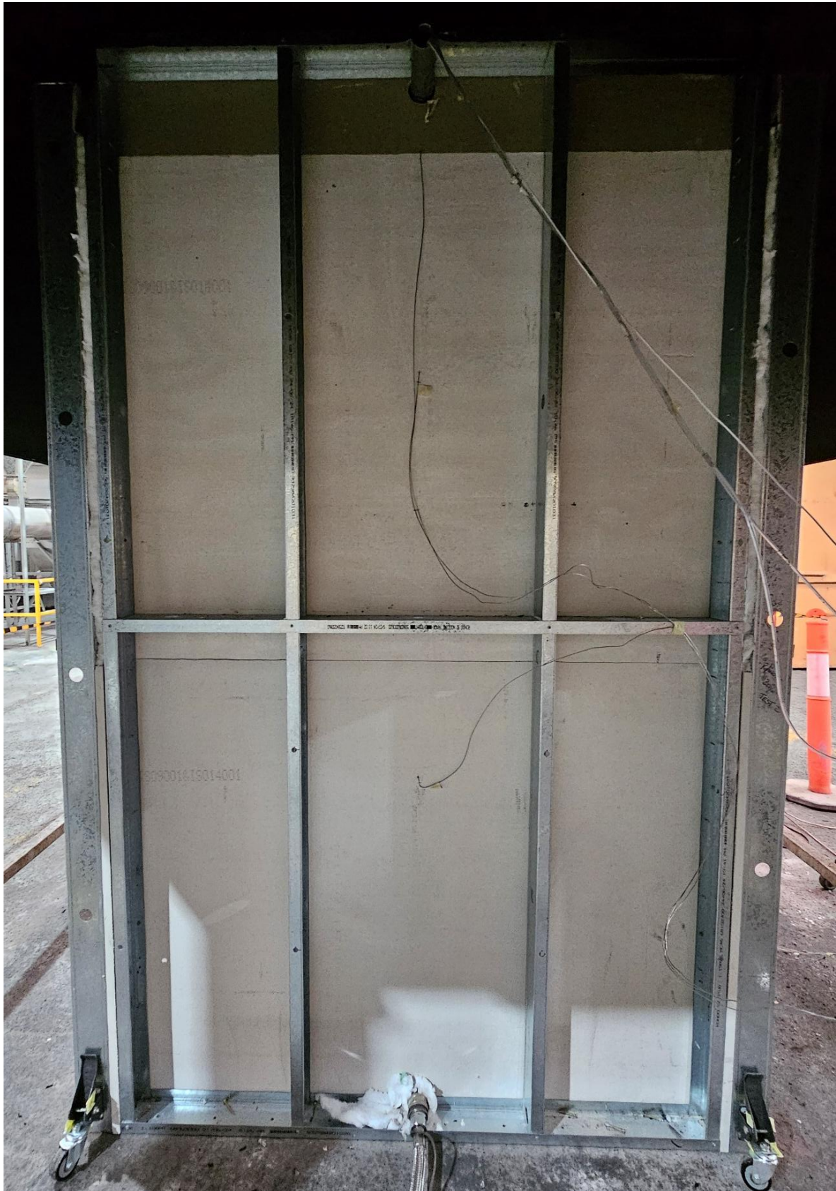
Figure 24 The specimen after the reaction to fire test – unexposed side
