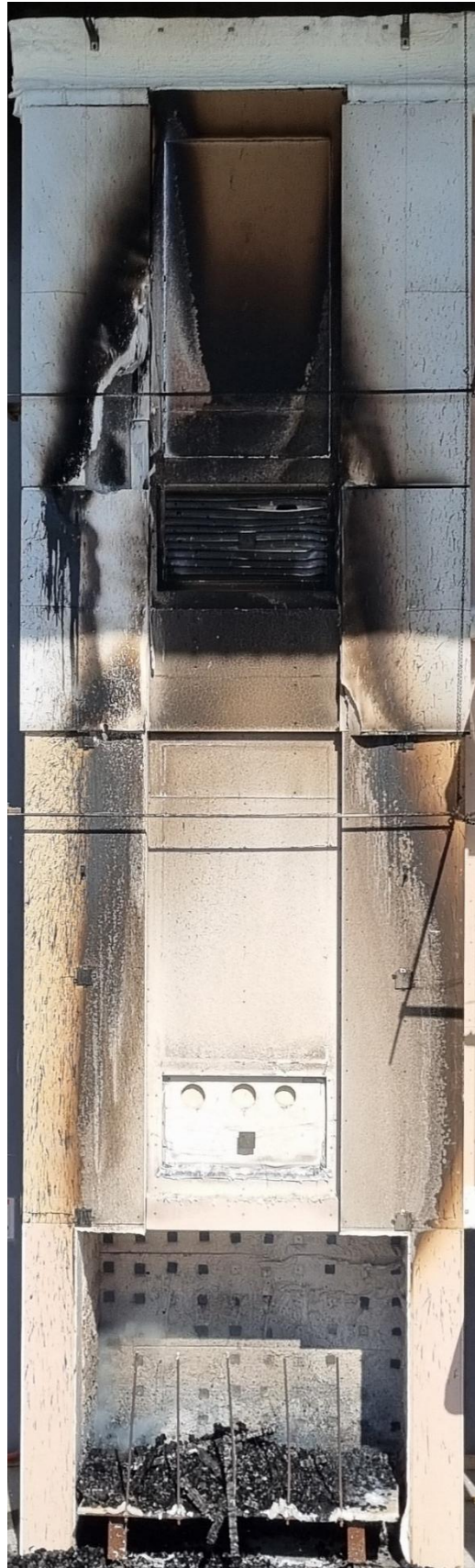
Figure 43 The external wall system on completion of the test – main wall
