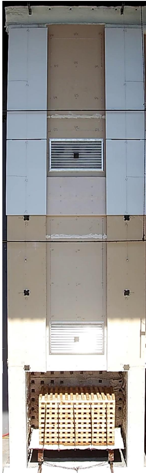
Figure 35 The external cladding system before the start of the test – main wall
