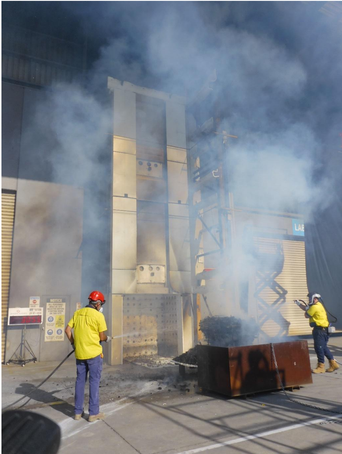
Figure 47 The external wall system during the test – after removal of the crib, 30 minutes 55 seconds after crib ignition
