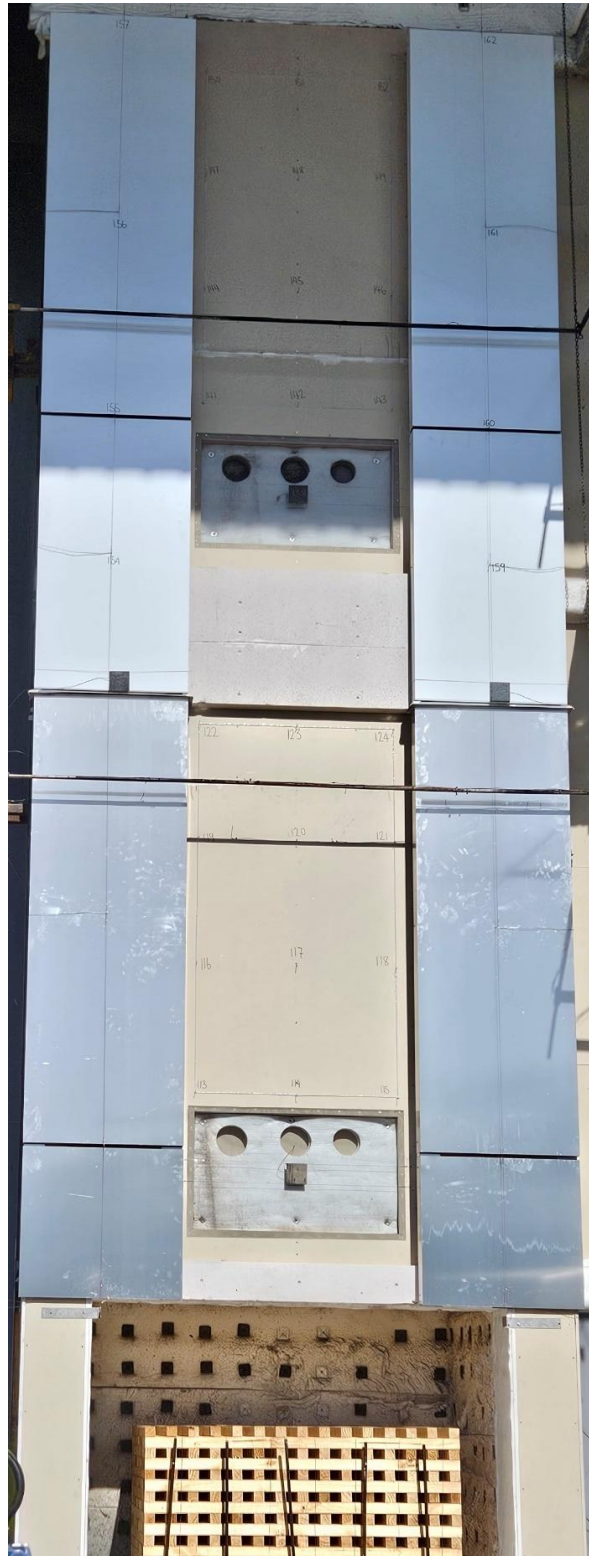
Figure 39 The external cladding system before the start of the test – main wall
