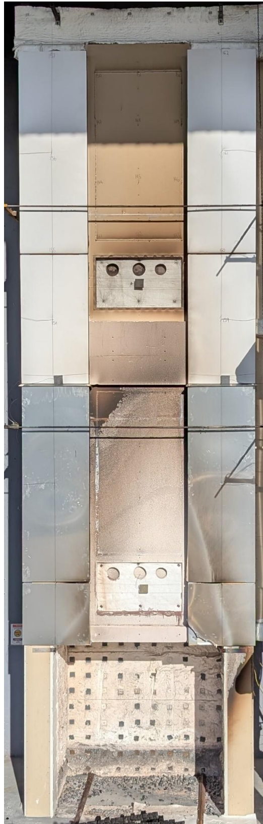
Figure 48 The external wall system on completion of the test – main wall
