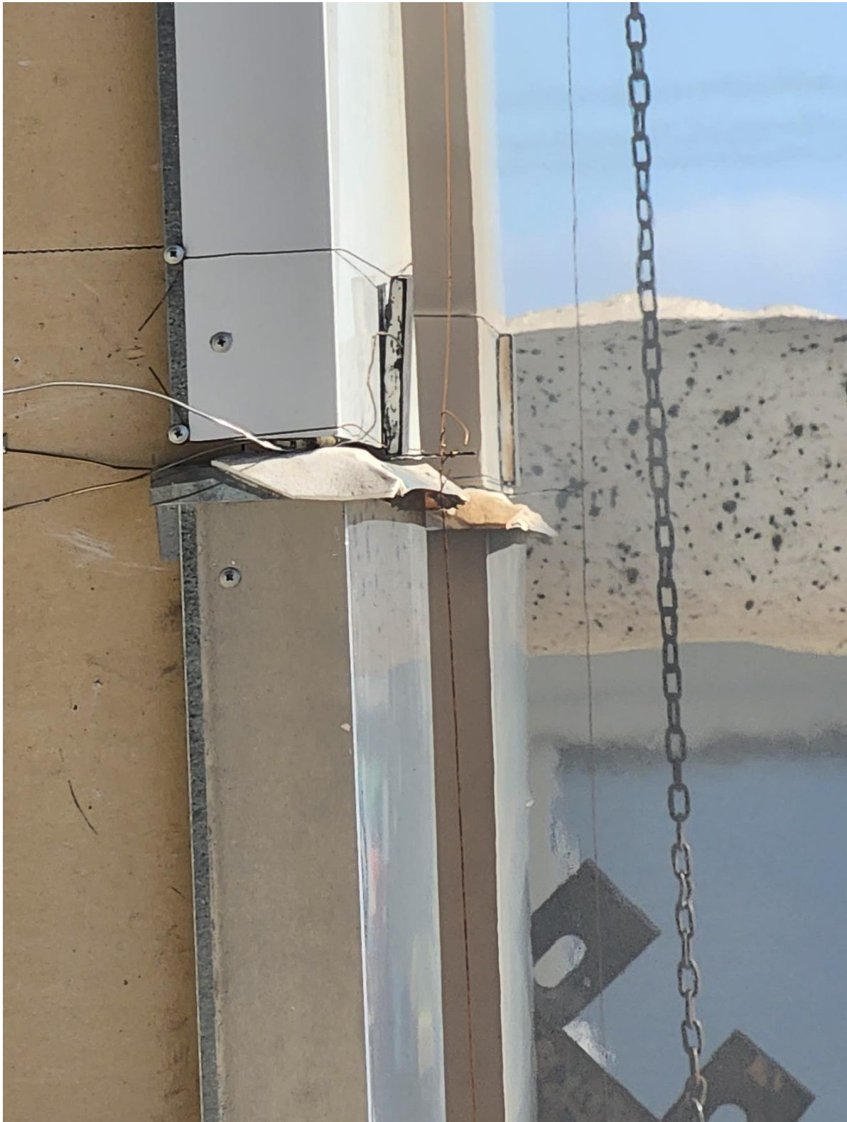
Figure 40 Flashing as installed – main wall
