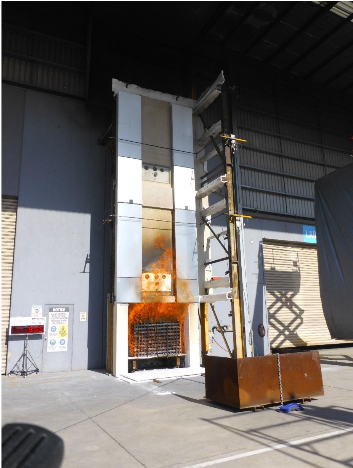
Figure 42 The external wall system during the test – 9 minutes 55 seconds after crib ignition
