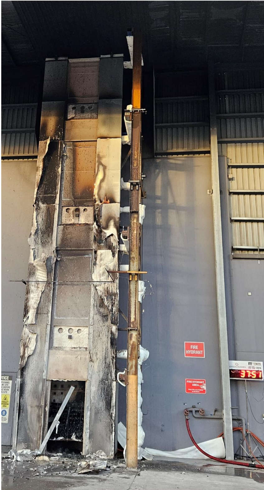
Figure 54 The external wall system – 7 minutes 51 seconds after crib was extinguished
