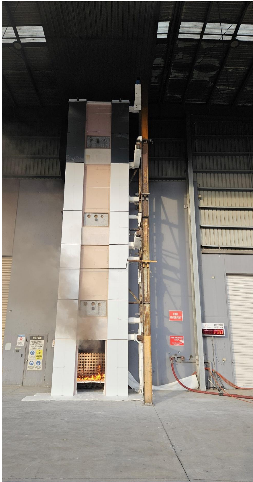
Figure 45 The external wall system during the test – 1 minute 30 seconds after crib ignition
