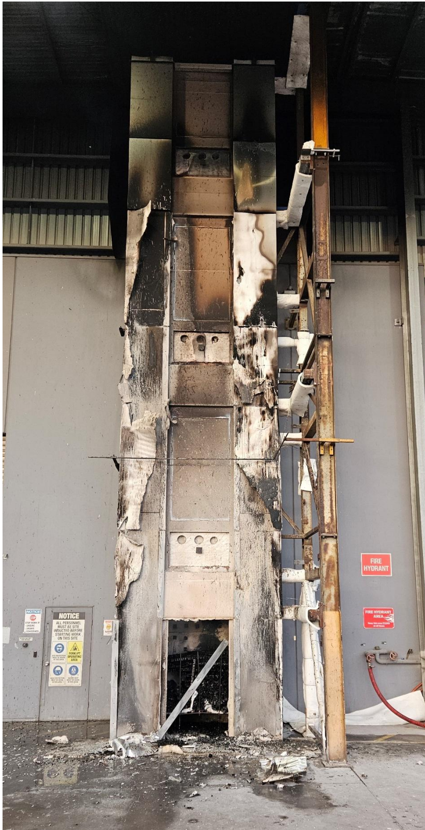
Figure 58 The external wall system on the completion of the test
