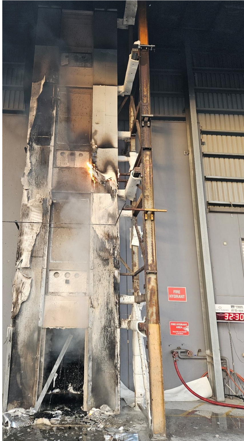
Figure 53 The external wall system – 2 minutes 30 seconds after crib was extinguished
