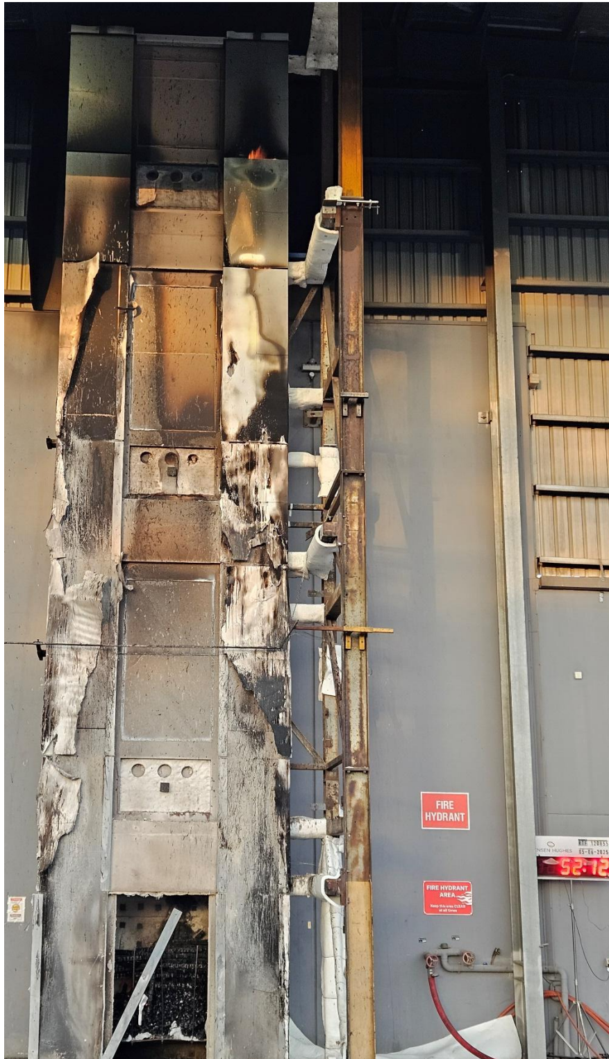
Figure 57 The external wall system – 22 minutes and 12 seconds after crib was extinguished
