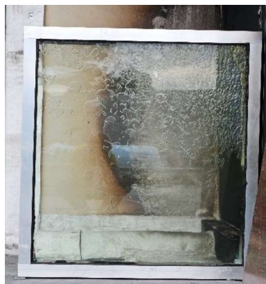
Figure 44 Post test condition of the ground level balustrade
