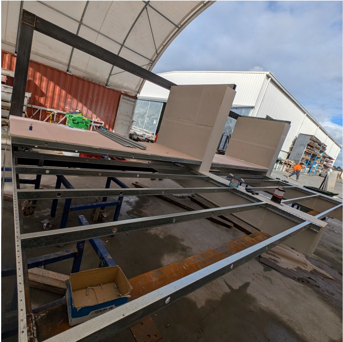
Figure 49 test jig during construction.
