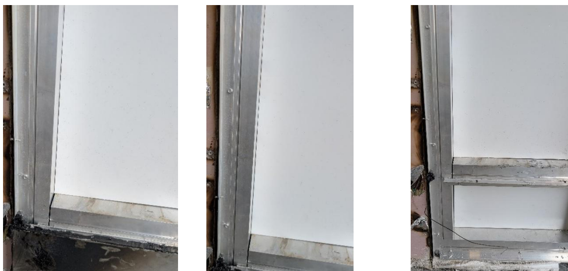
Figure 48 Post test condition of the ACP back pan.
