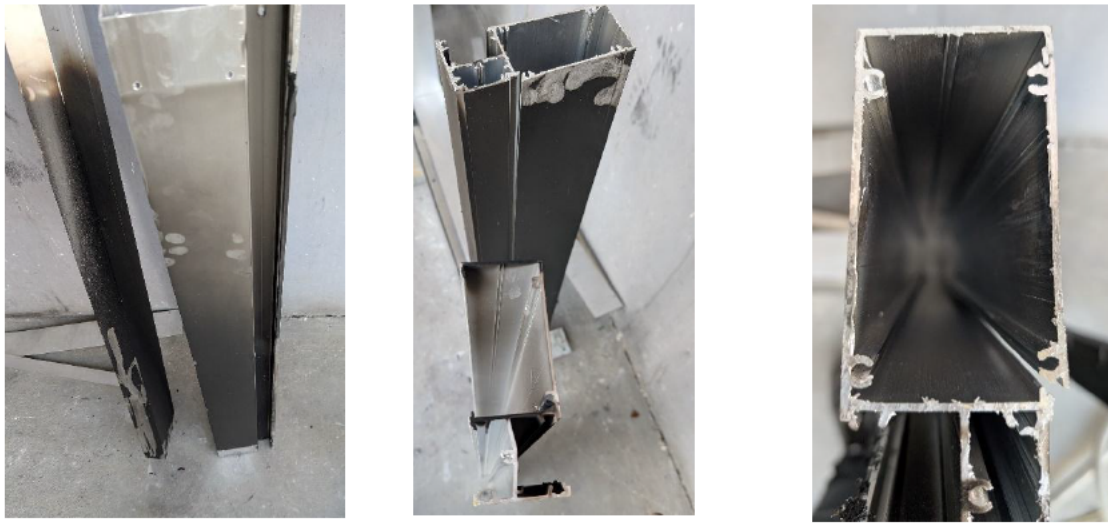
Figure 45 Post test condition of the ground level balustrade.
