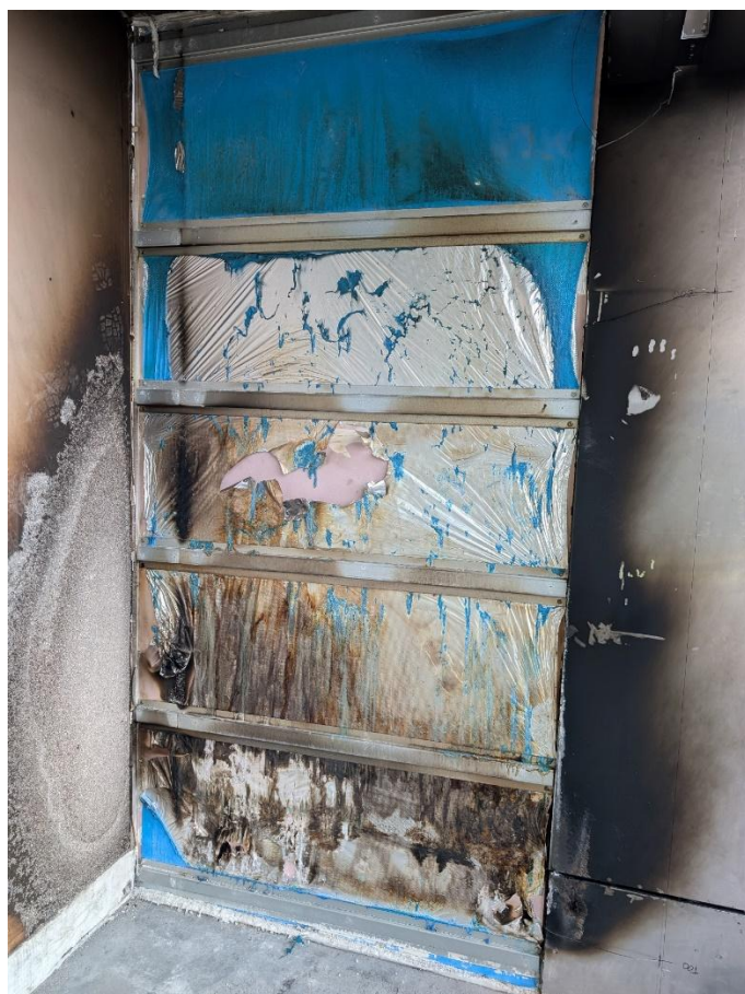
Figure 47 Post test condition behind the MgO board.
