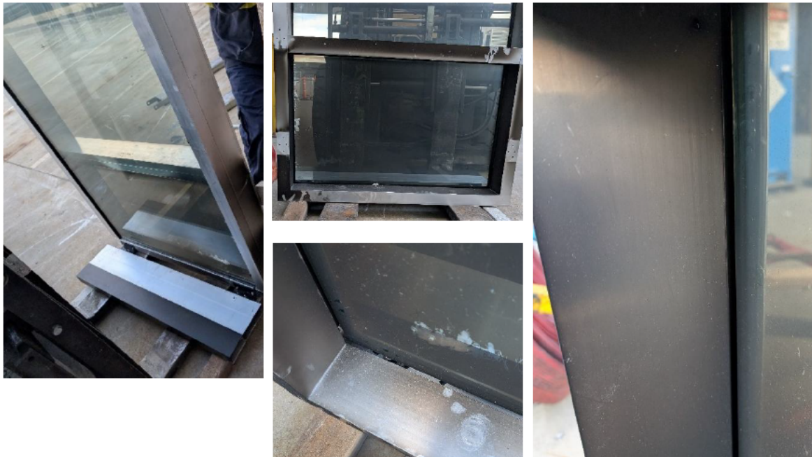
Figure 46 Post test condition of level 1 balustrade.
