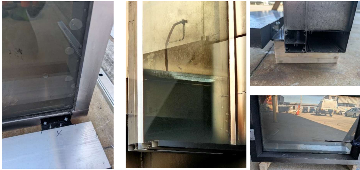
Figure 45 Post test condition of level 1 balustrade
