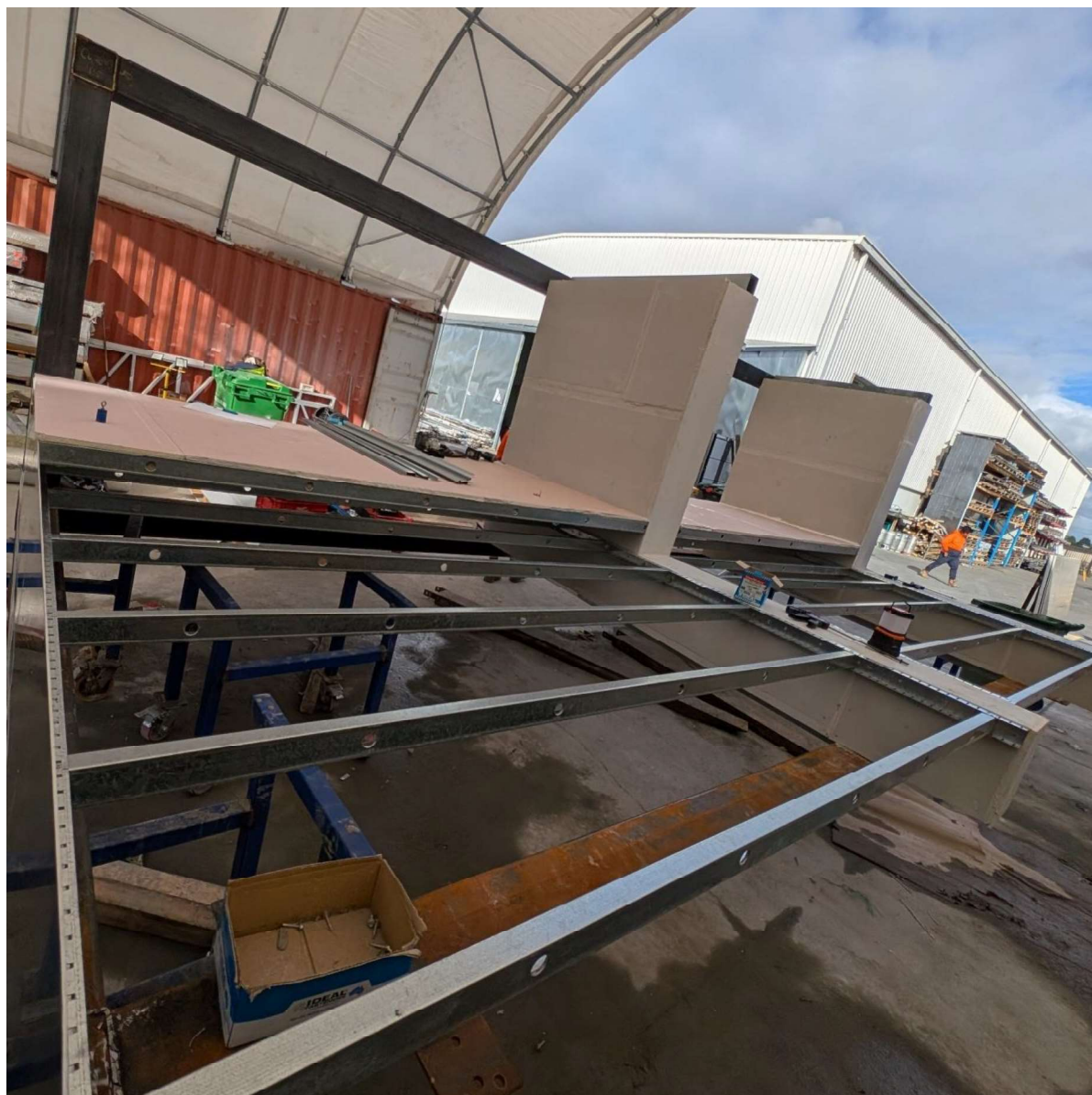
Figure 48 test jig during construction
