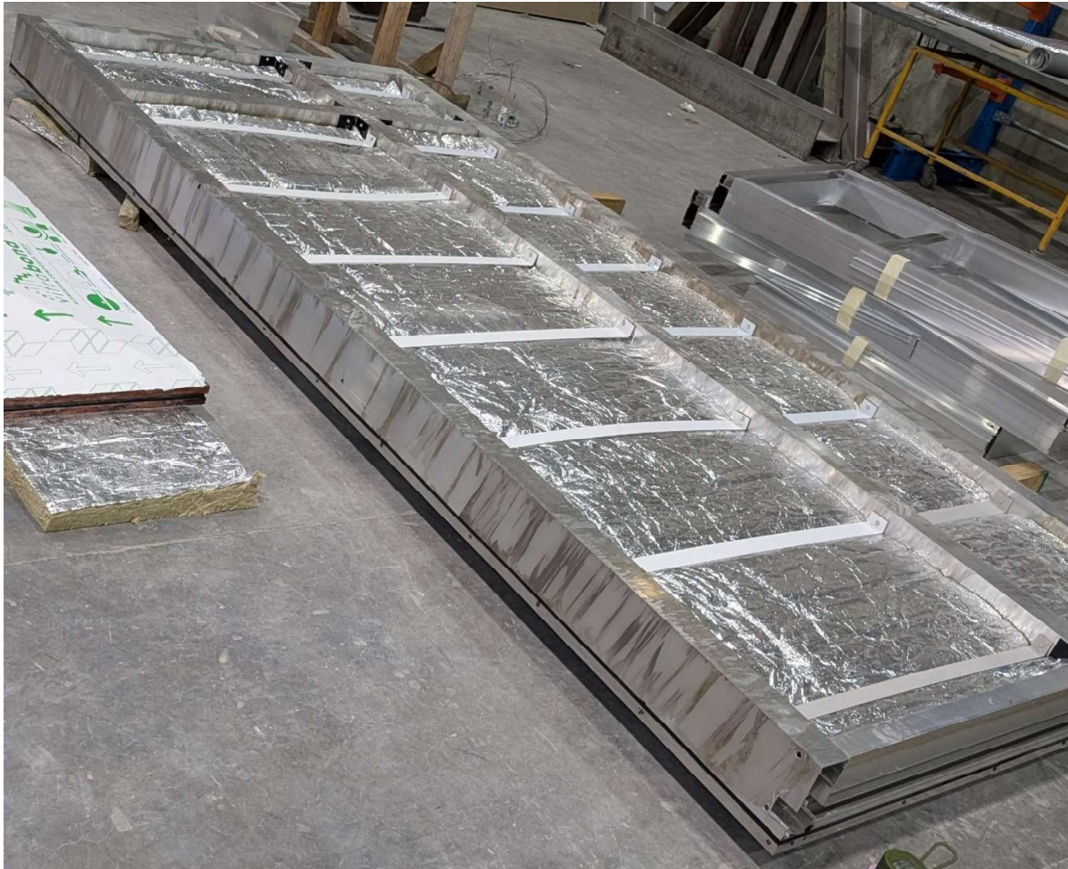
Figure 49 unexposed side of ACP curtainwall module
