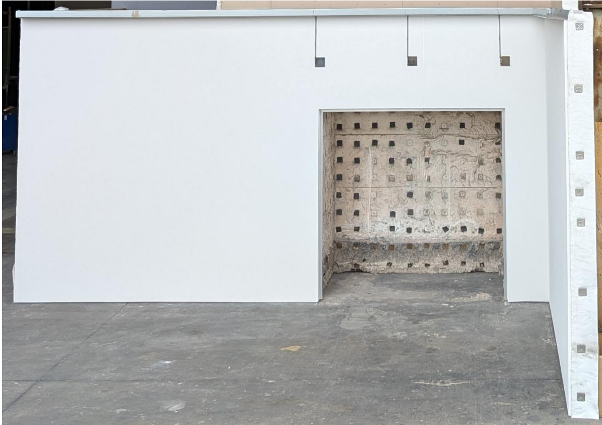
Figure 24 The wall system before the start of the test – main wall
