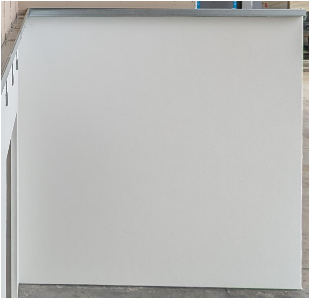
Figure 25 The wall system before the start of the test – wing wall
