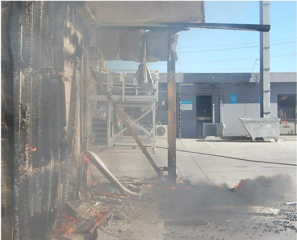
Figure 39 The wall system on completion of the test – wing wall
