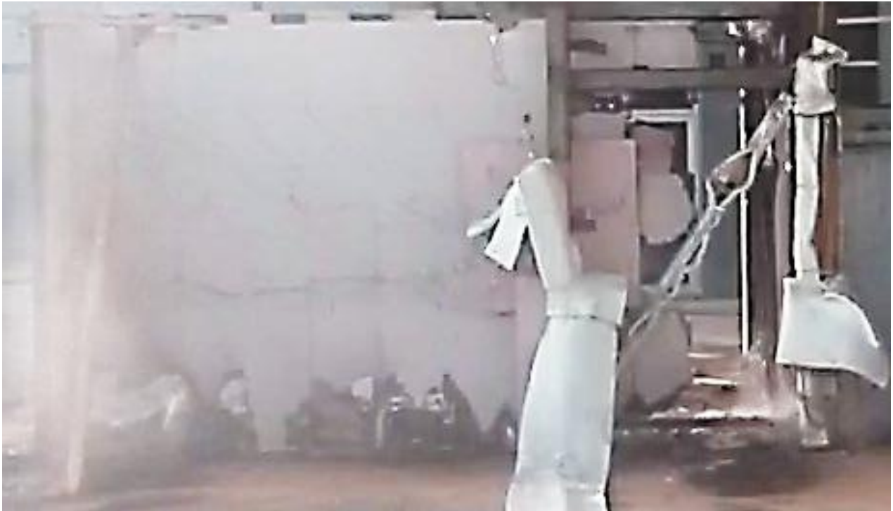
Figure 53 The wall system on completion of the test – unexposed wing and return wall
