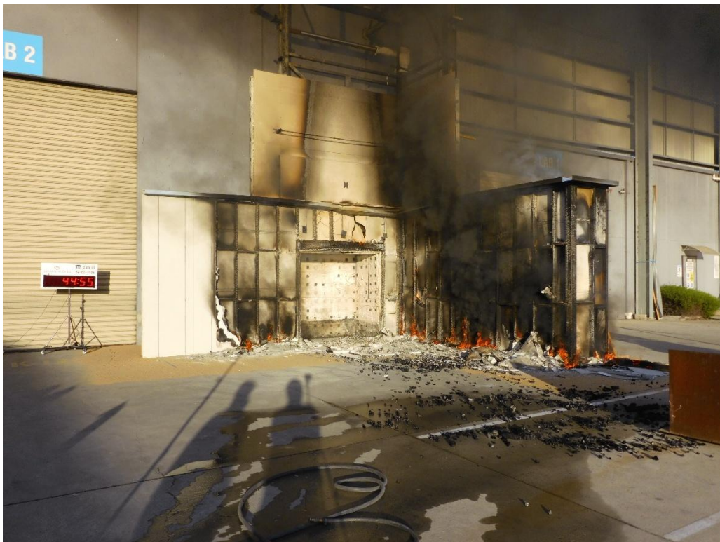
Figure 48 The wall system during the test – 44 minutes 55 seconds after crib ignition
