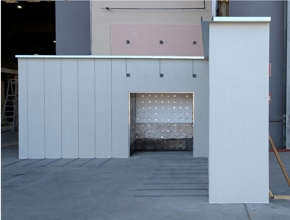
Figure 37 The wall system before the start of the test
