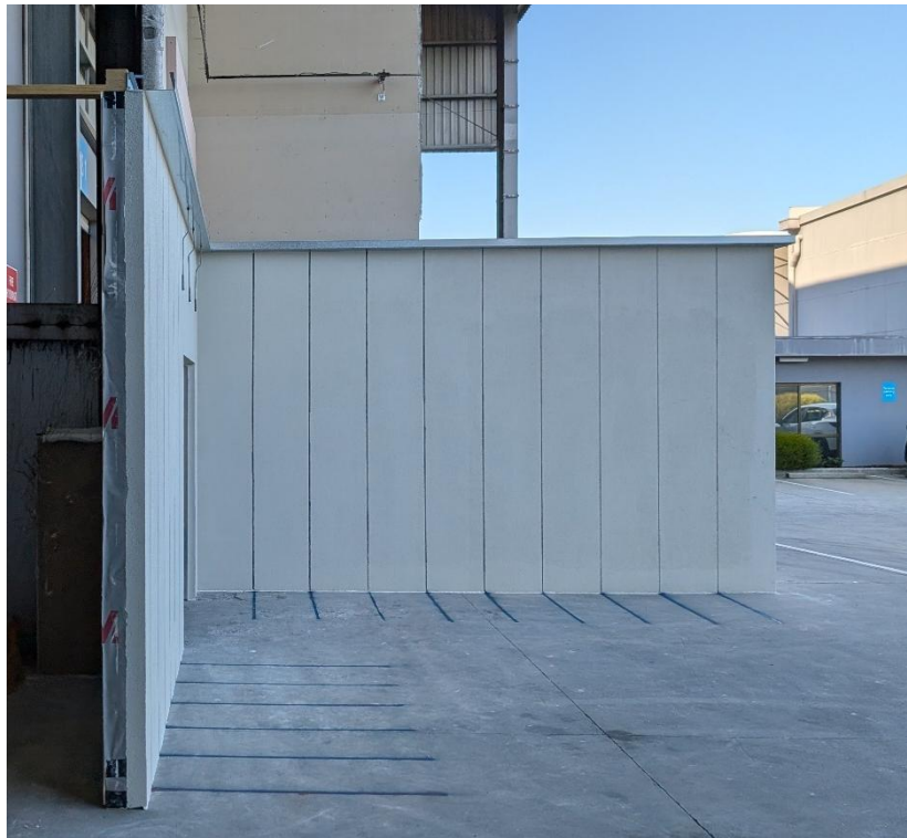
Figure 38 The wall system before the start of the test
