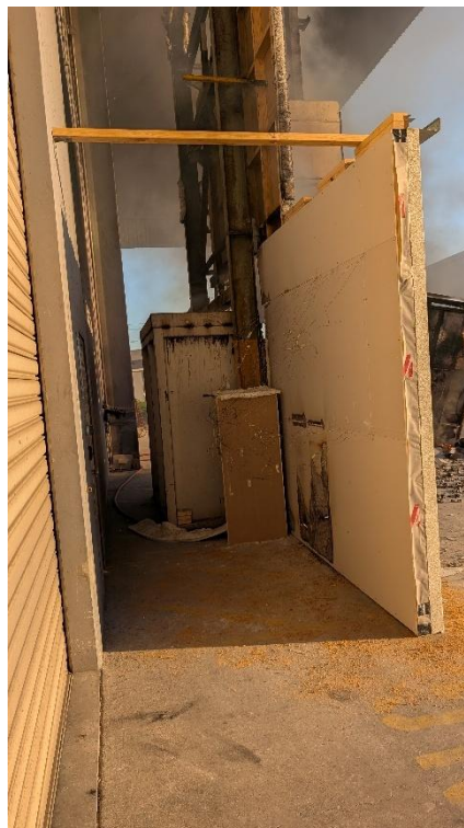
Figure 54 The wall system on completion of the test – unexposed main wall face
