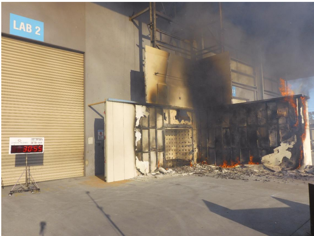
Figure 46 The wall system during the test – after removal of the crib, 30 minutes 55 seconds after ignition of crib
