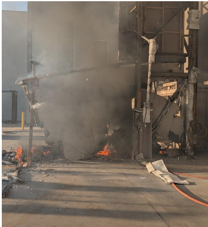
Figure 55 The wall system on completion of the test – unexposed wing and return wall
