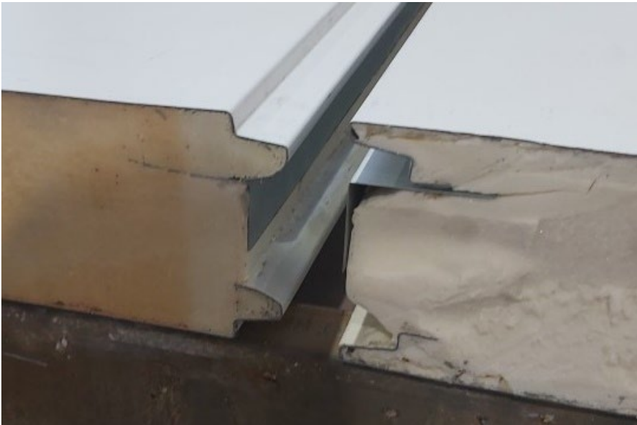
Figure 2. ISP-01 (PIR) sandwich panel joint profile with Steel "L" flashing installed to edge joints.
