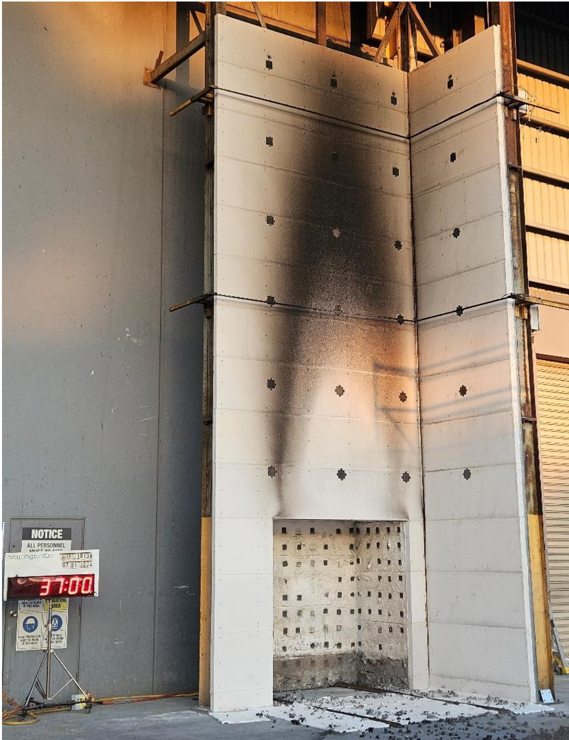
Figure 23 The external wall system during the test – 37 minutes after crib ignition
