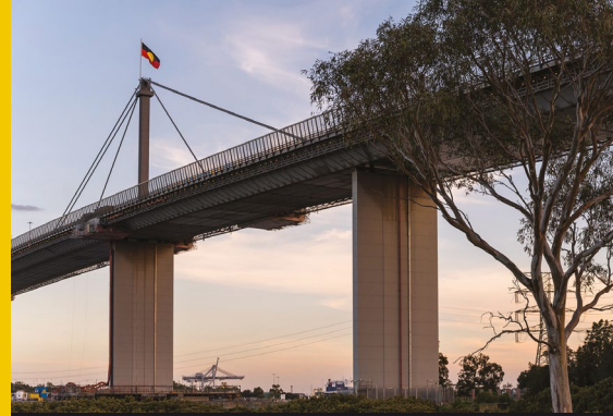
Aboriginal Flag flying permanently on the West Gate Bridge
